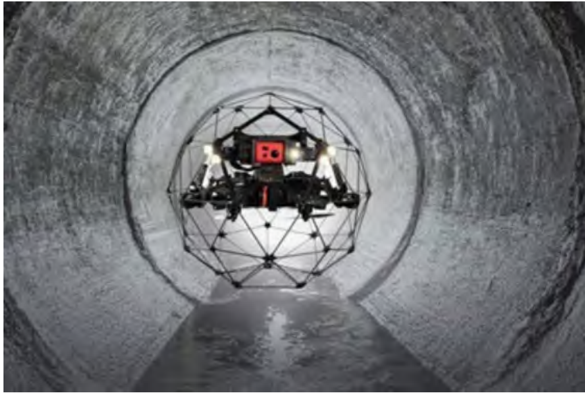
Figure 5. UAS Inspection of Large Pipe. Source: MDOT
