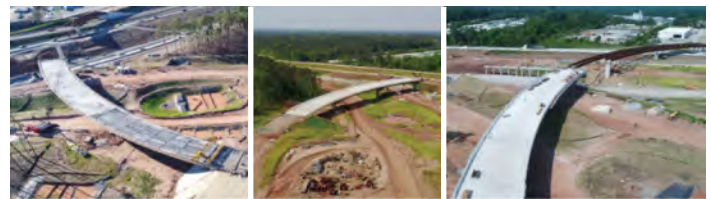
Figure 5. Construction progress on a flyover bridge
