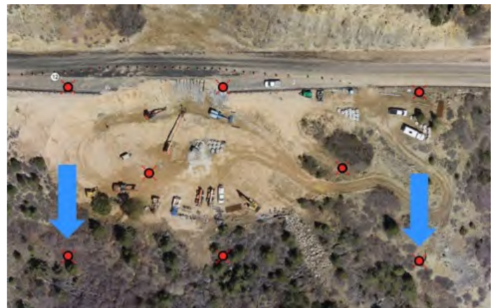
Figure 9. GCPs placement (Image courtesy of UDOT)
