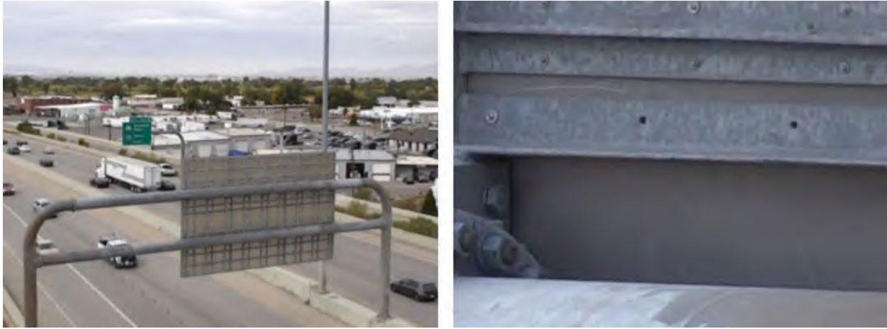
Figure 6. UAS Overhead Sign Inspection. Source: UDOT
