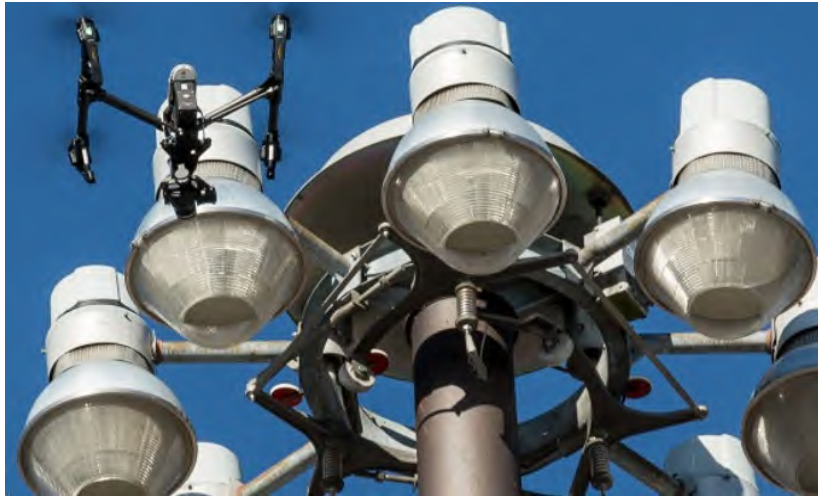
Figure 1. UAS Inspecting HMLP. Source: NJDOT
